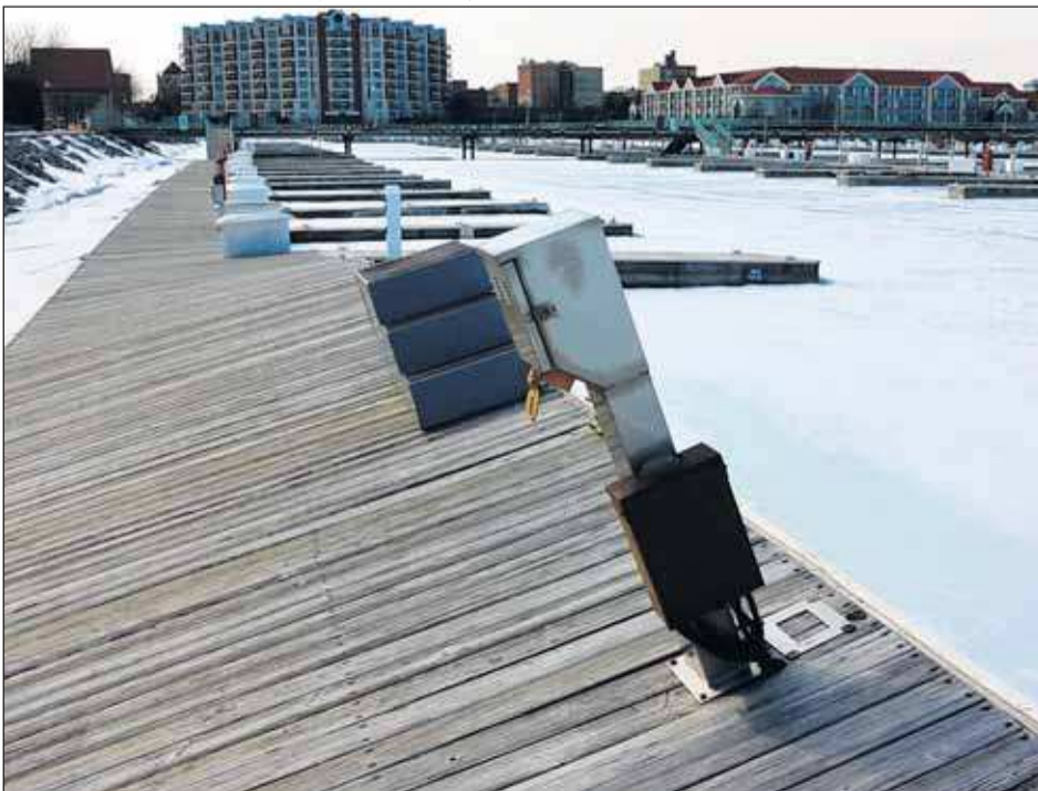
GREGORY SHAVER gregory.shaver@journaltimes.com Ice has moved and pushed parts of the docking at Reef Point Marina out of the water in this photo from Wednesday. The melting of that ice is at hand: Today the forecast calls for rain instead of snow, the highs for the four days to follow are all above freezing, and the highs for Sunday and Monday are forecast to be 54 and 50, respectively.
